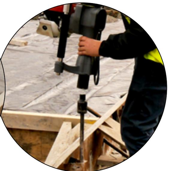
Unlike hammering the form stakes in, using the Drive Shim prevents mushrooming and splintering which can occur over time. The long-term cost saving of keeping these form stakes usable on multiple jobs is very positive for the industry.
