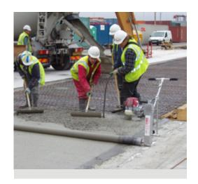
The RT6 Rotoscreed Mini Striker is ideal for small concrete pours and is powered by a Honda GX35 unit providing ample power and unparalleled reliability.
