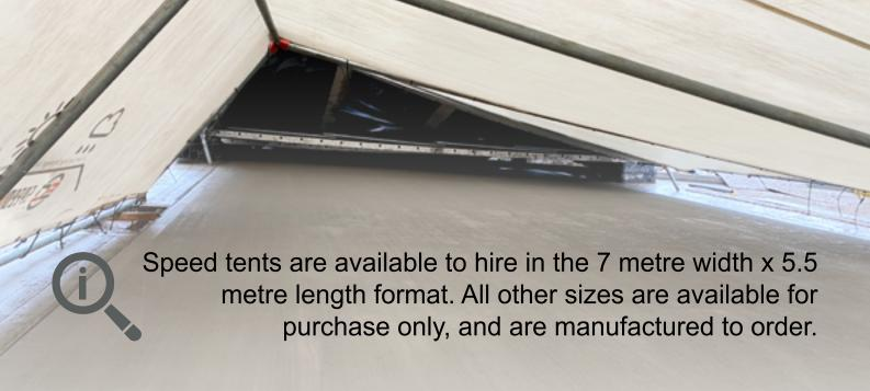
The dimension tolerance allows for sufficient overlap to prevent water ingress onto the slab surface. For example a 7 x 5.5 metre tent will cover a bay width of 6 meters and a linear length of 5 meters.
