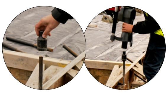
Unlike hammering the form stakes in, using the Drive Shim prevents mushrooming and splintering which can occur over time. The long-term cost saving of keeping these form stakes usable on multiple jobs is very positive for the industry.
