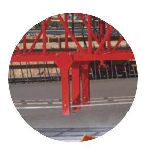
28" (71 cm) height from top of the deck to slab vertically adjustable end frames from 16" - 36" (40.6 - 91.4 cm) from the top of the deck to slab optional.
